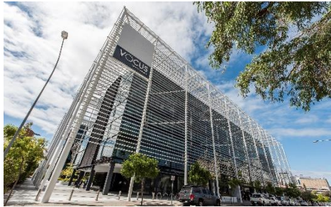
WorkZone West 202 Pier Street, Perth
