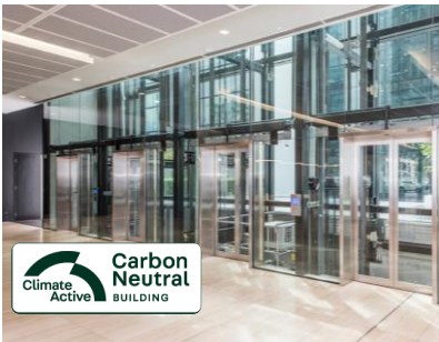
WorkZone West 6 Star NABERS Energy and Carbon Neutral certification
