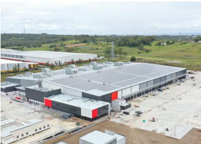
The Sydney Ocado customer fulfilment centre is expected to open in early FY24.
