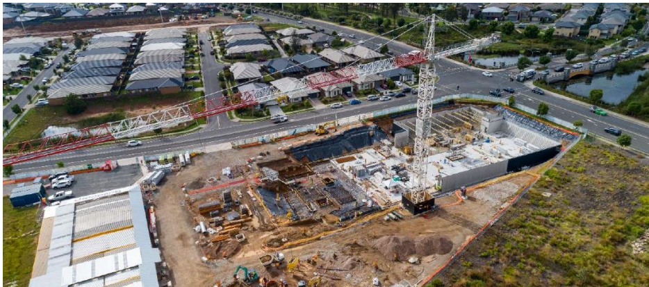
HCW development in progress – The George Hospital Camden Stage 1 (NSW)
