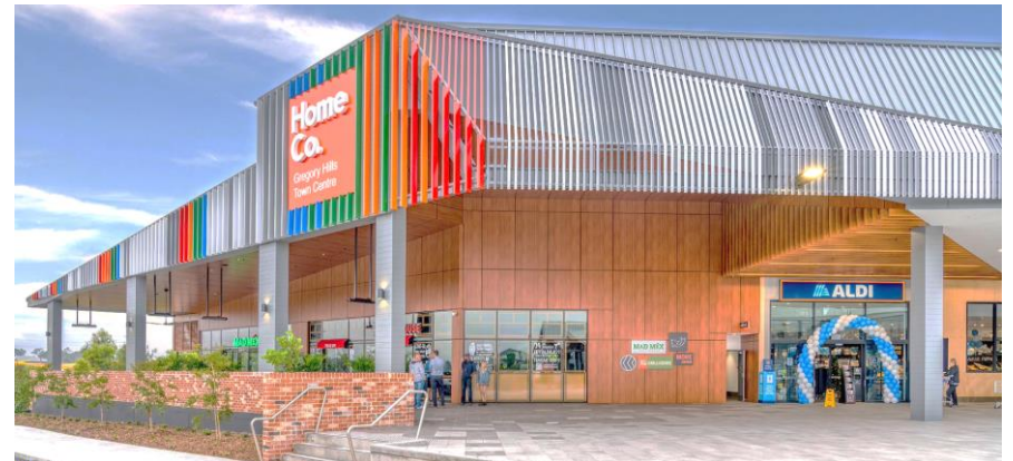
HDN development completed 1H FY22 – Gregory Hills Town Centre (NSW)
