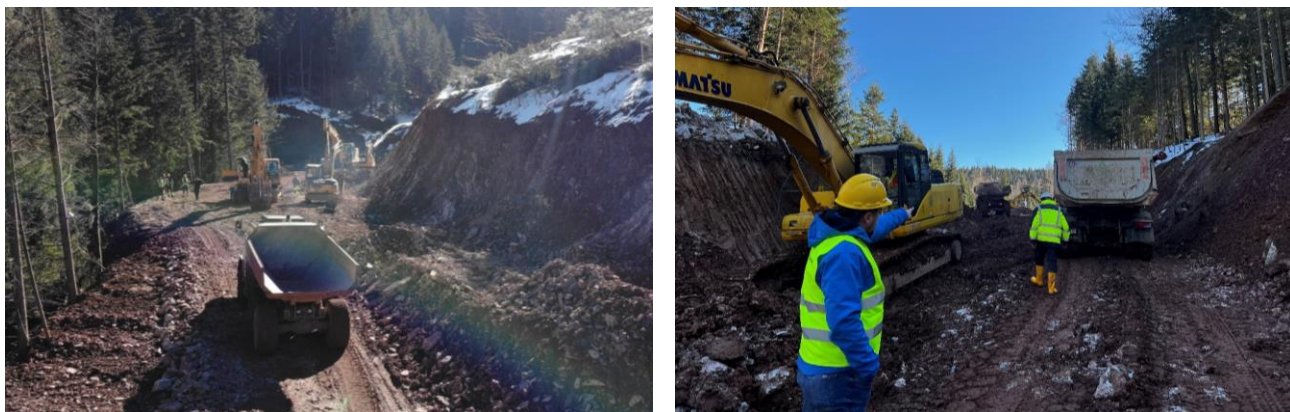
Figure 1: Site clearing and construction of the access road to the lower and upper portals
