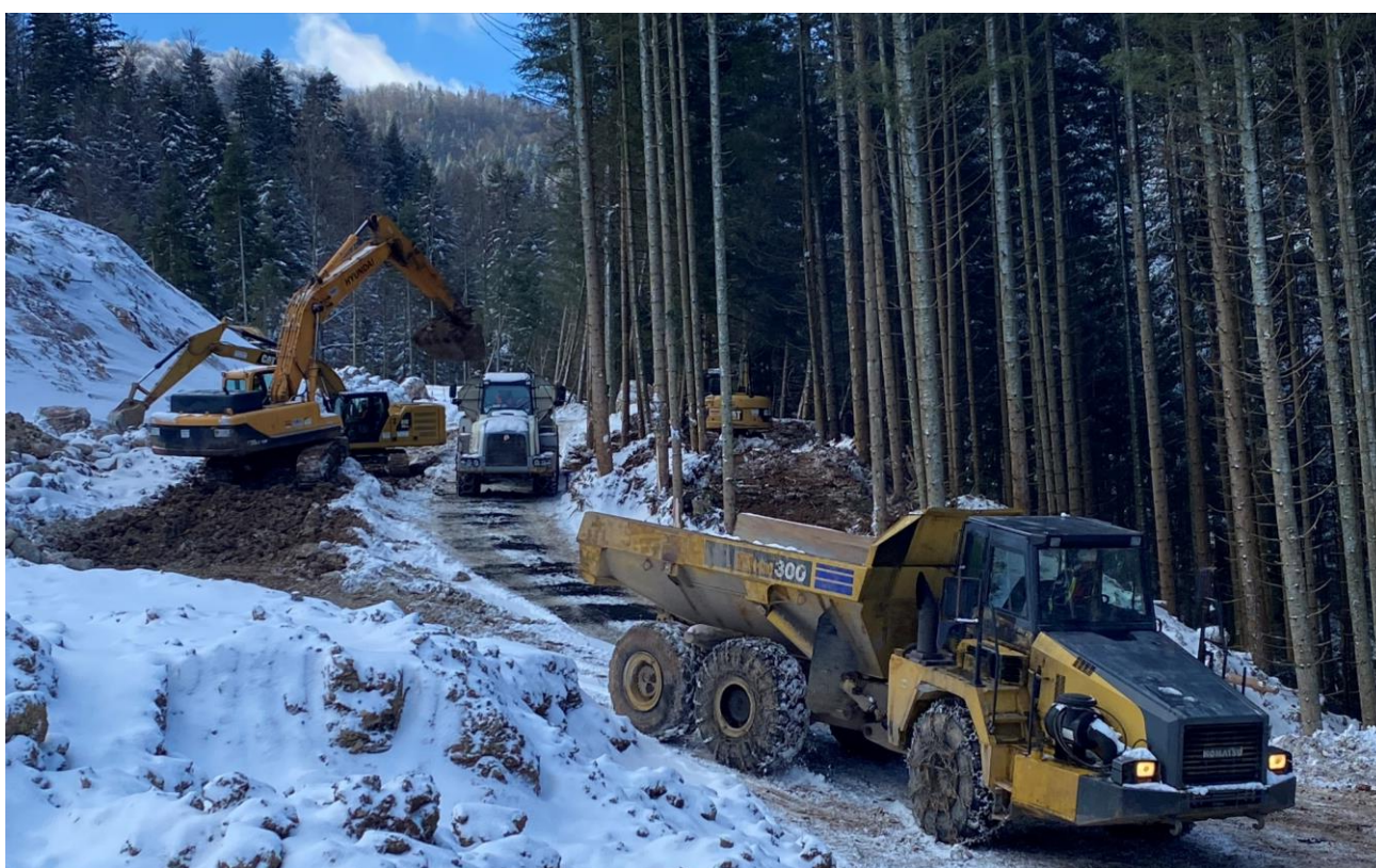
Figure 2: Site clearing and construction of the access road to the lower and upper portals
