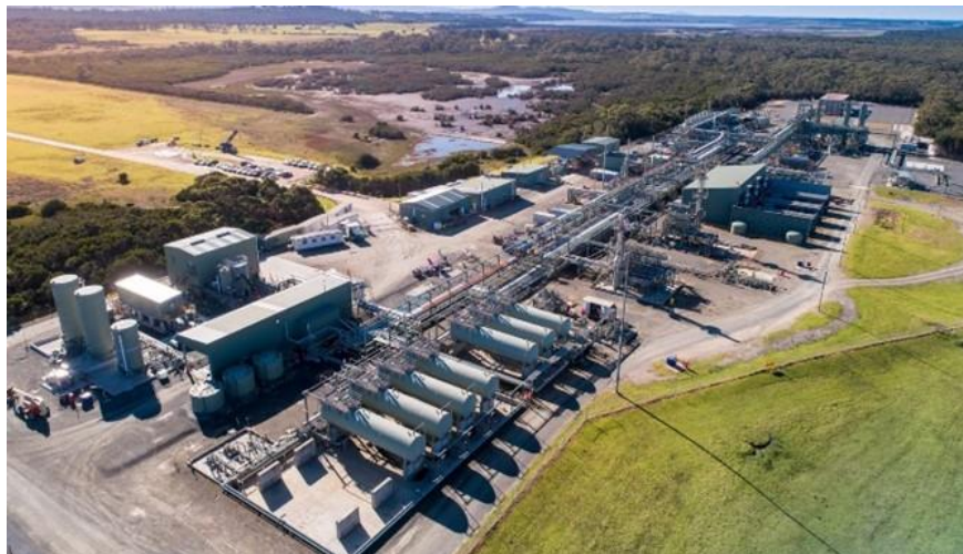
Orbost Gas Processing Plant, owned and operated by APA
