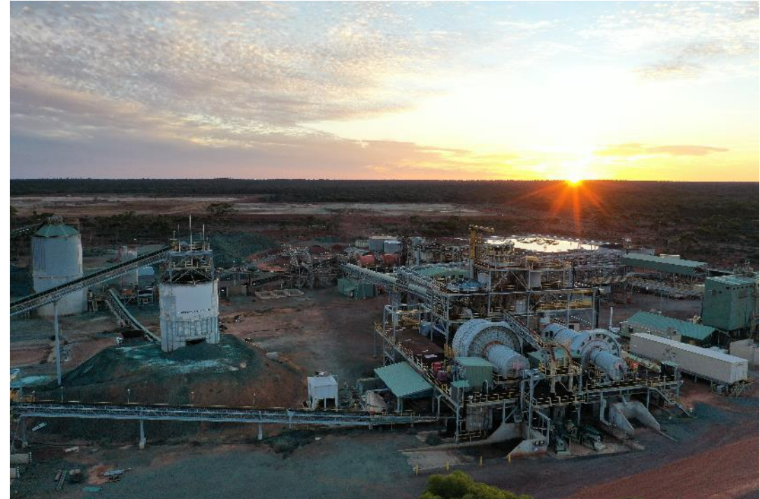
Black Swan 2.2Mtpa milling circuit Plans to refurbish and de-rate to 1.1Mtpa throughput
