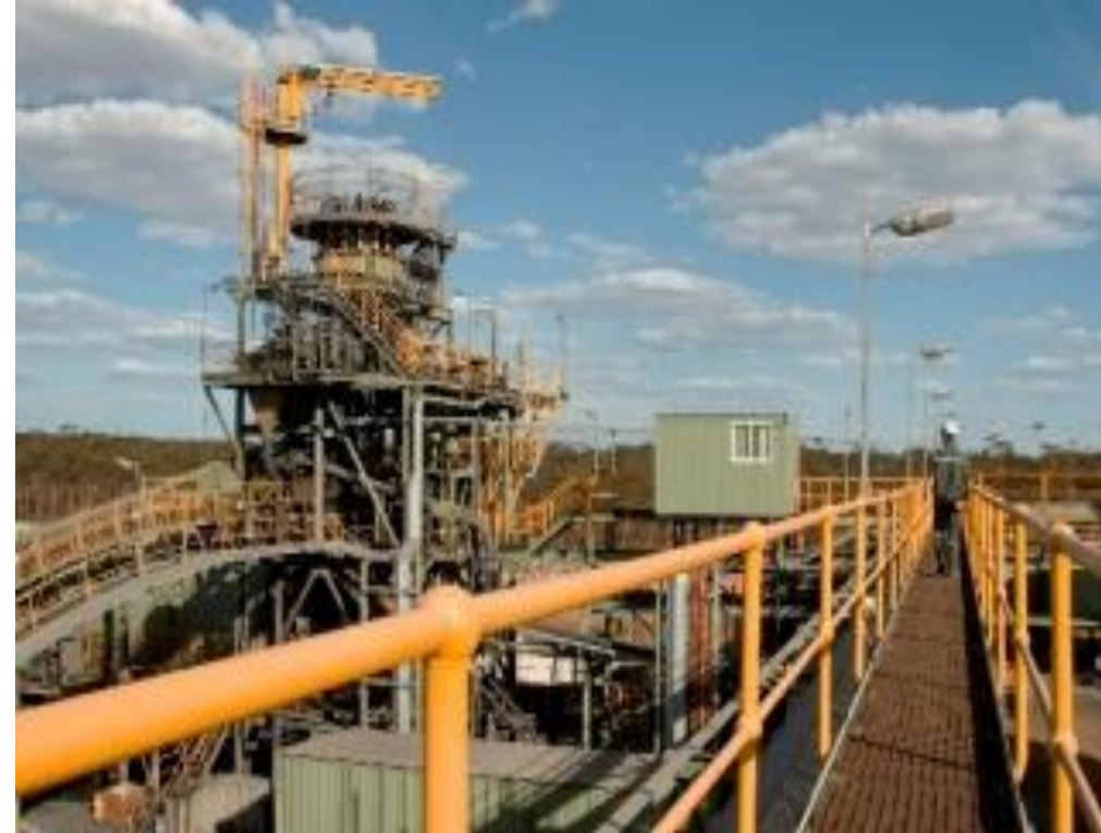
Lake Johnston 1.5Mtpa processing plant
