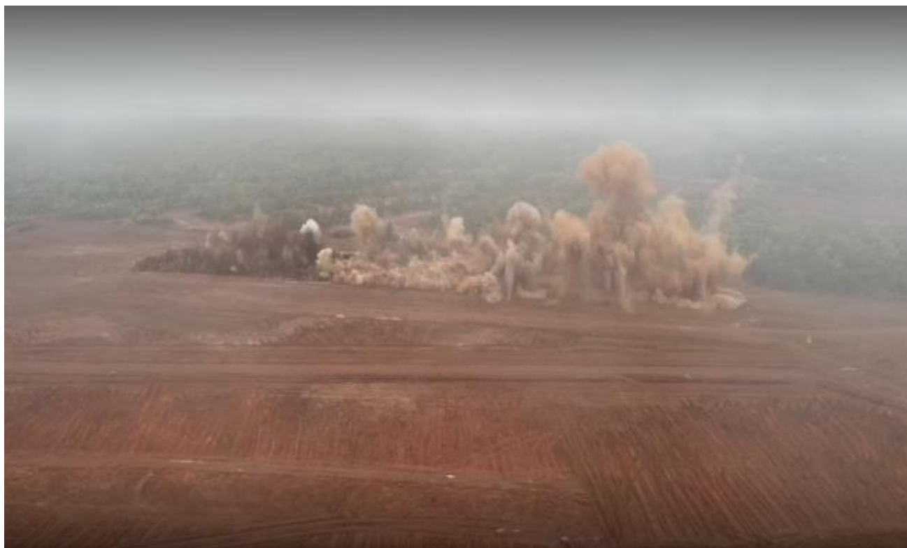
Figure 2: Aurelia breaks ground with the first blast in the box cut
