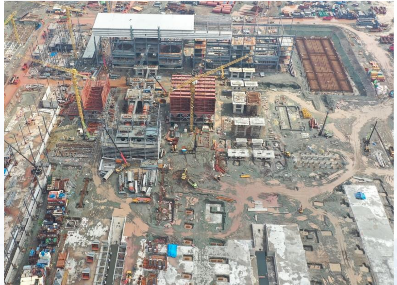
An aerial image of ONI construction progress within the IMIP
