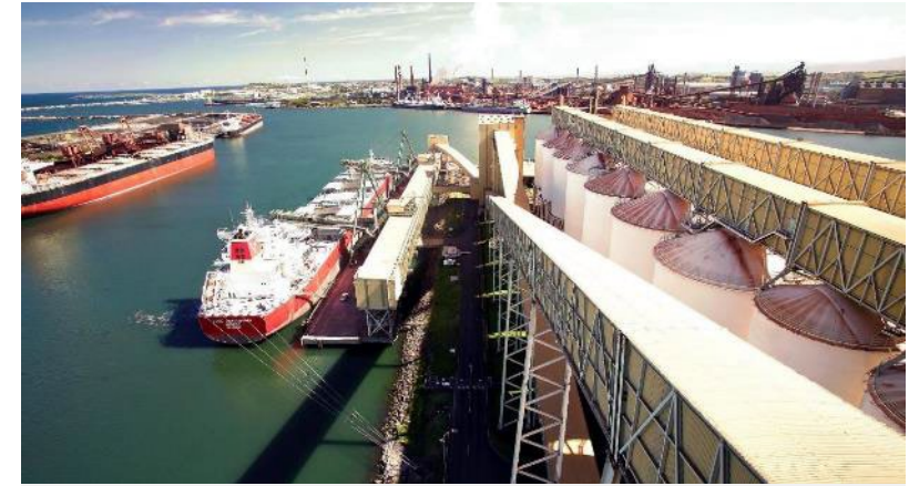
GrainCorp bulk port terminal, Port Kembla, NSW
