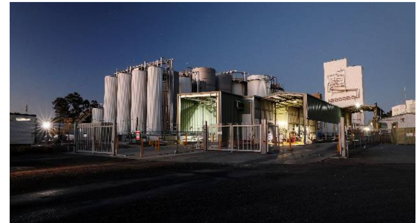
GrainCorp oilseed crush plant, Numurkah, VIC
