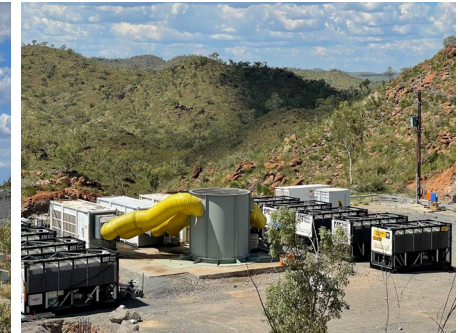
6MW Chiller Plant
