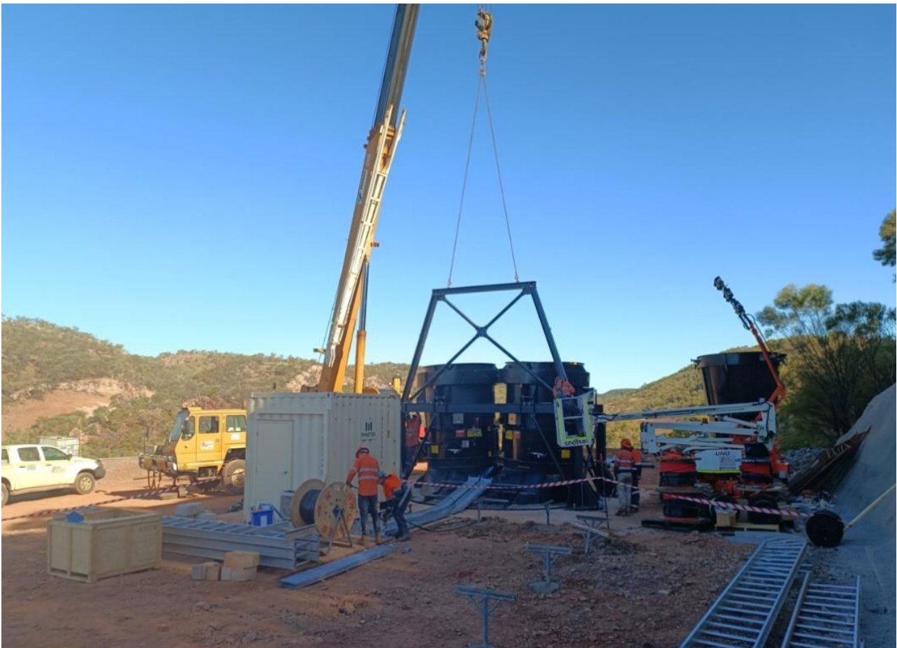
Installation of ESS ventilation infrastructure at Capricorn Copper
