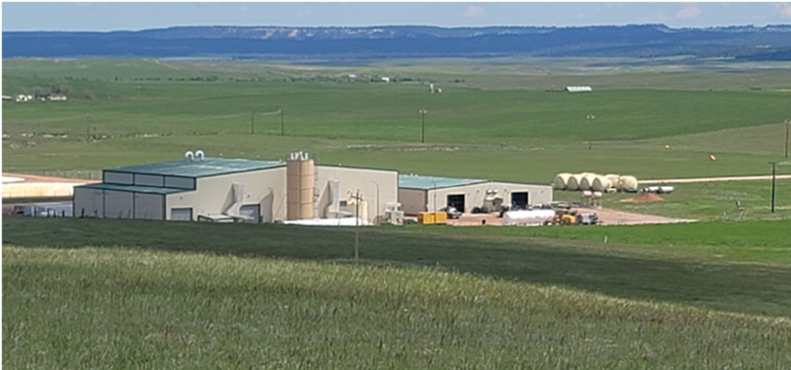
Image 1: The Ross Process Plant at the Lance Projects, Wyoming USA
