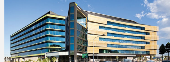
Energex House, Brisbane
