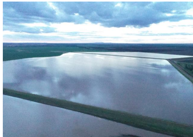
Water storage increase of 4,142 ML was completed in 2020, February 2022.
