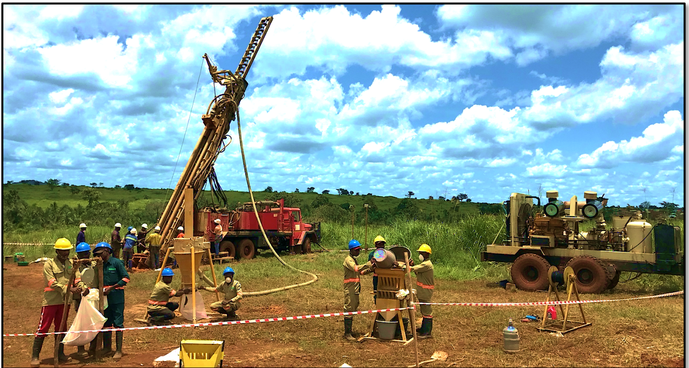
Figure 1 - RC Rig and Drill Crew at Kebigada South-East
