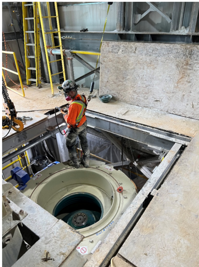
Figure 3: Installation of the HP 300 and preparation for HP 400
