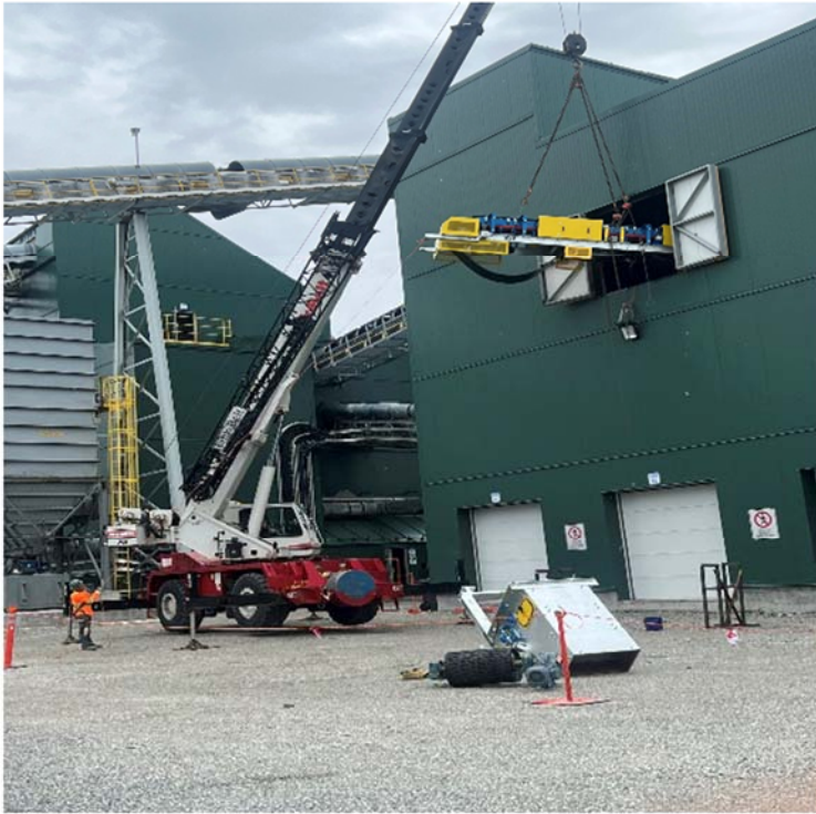
Figure 4: Installation of the third ore sorter conveyors
