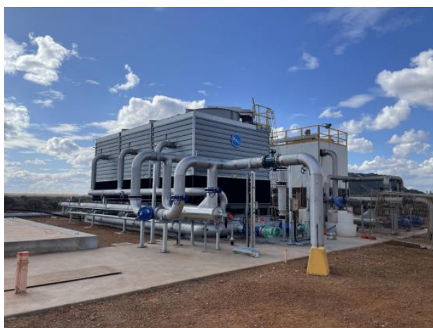
3.2MW bulk air coolers and chiller plant installed as part of the second stage surface cooling plant upgrade. Additional chilled air will be distributed to XE orebody to further improve underground operating conditions.
