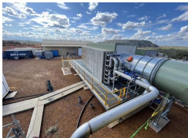
3.2MW bulk air coolers and chiller plant installed as part of the second stage surface cooling plant upgrade. Additional chilled air will be distributed to XE orebody to further improve underground operating conditions.
