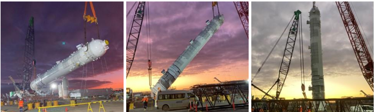
Waitsia Stage 2 CO 2 absorber lift
