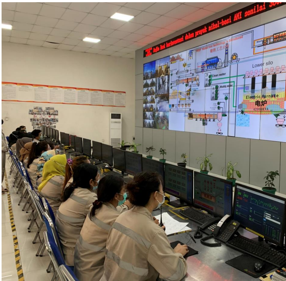
Control room at ANI
