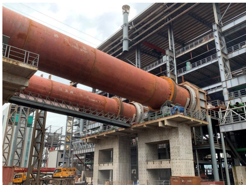
Rotary kilns at ONI under construction
