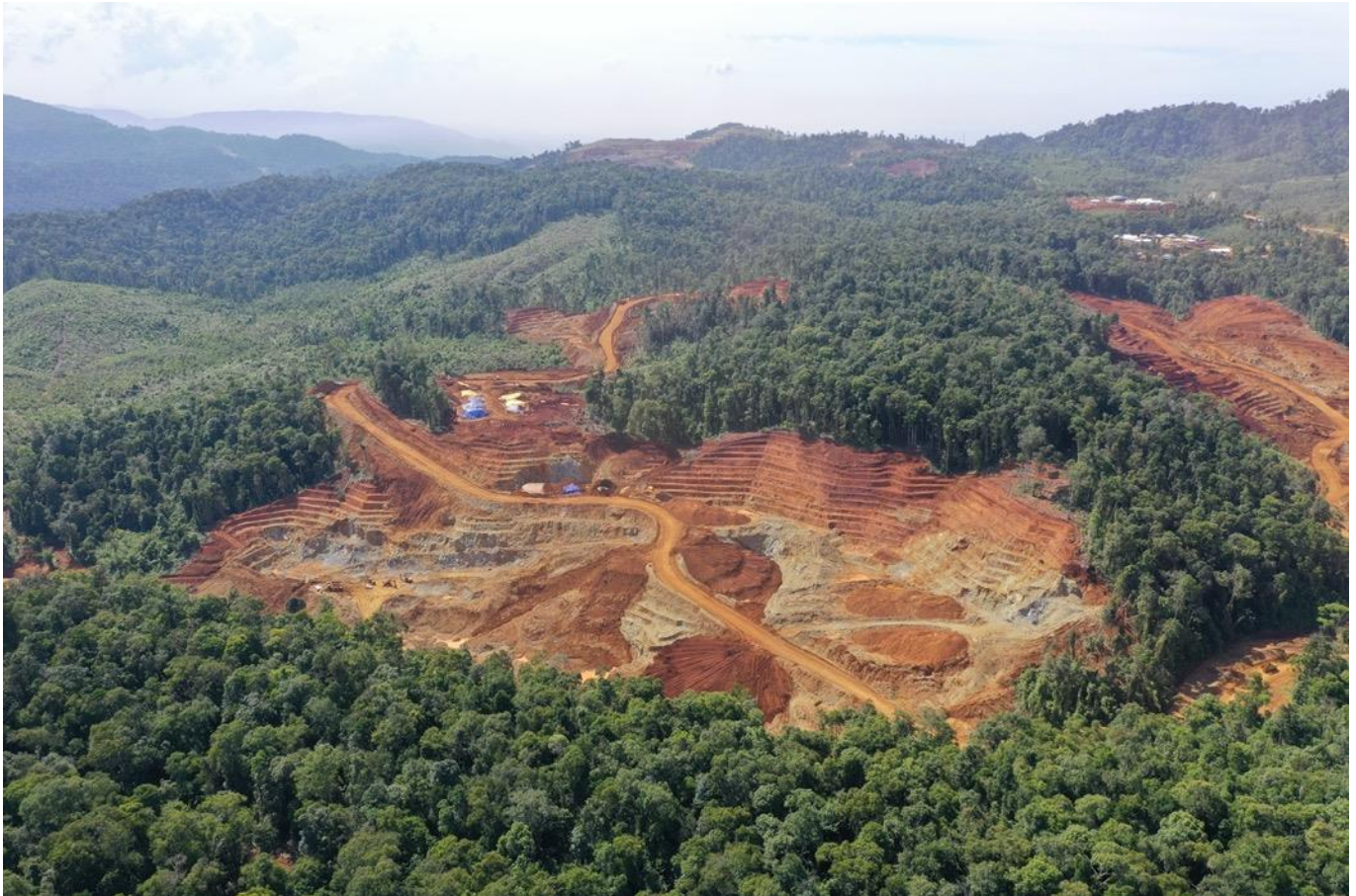
Mine operations at 3mtpa capacity. Central in foreground, Bete Bete in background.
