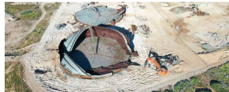
Thevenard Island decommissioning
