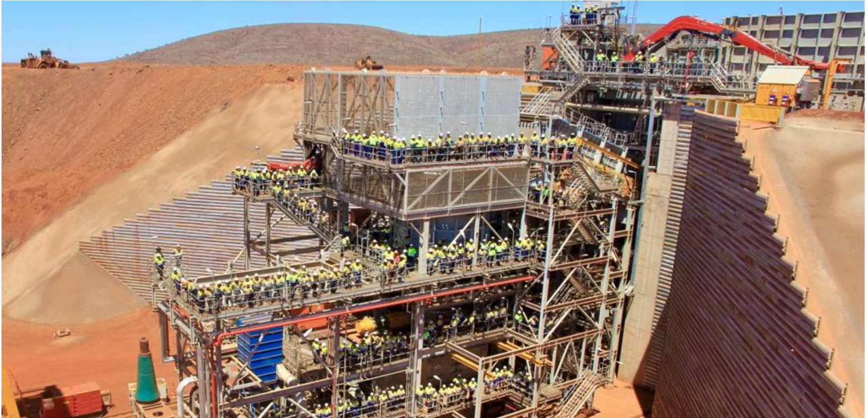
Rio Tinto's Western Turner Syncline Phase 2 Project, Tom Price, Western Australia.
