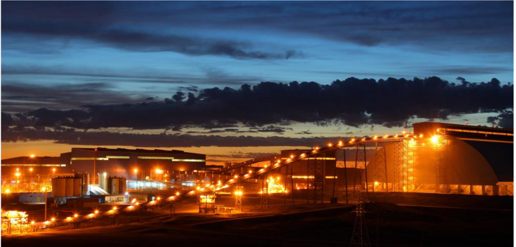
Rio Tinto's Oyu Tolgoi Underground Project, South Gobi region, Mongolia. Image courtesy of Rio Tinto.
