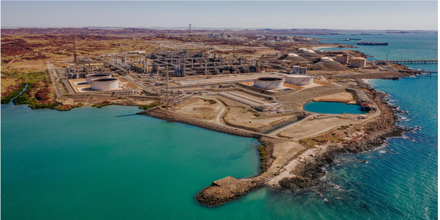
Woodside-operated Karratha Gas Plant, Karratha, Western Australia. Image courtesy of Woodside.
