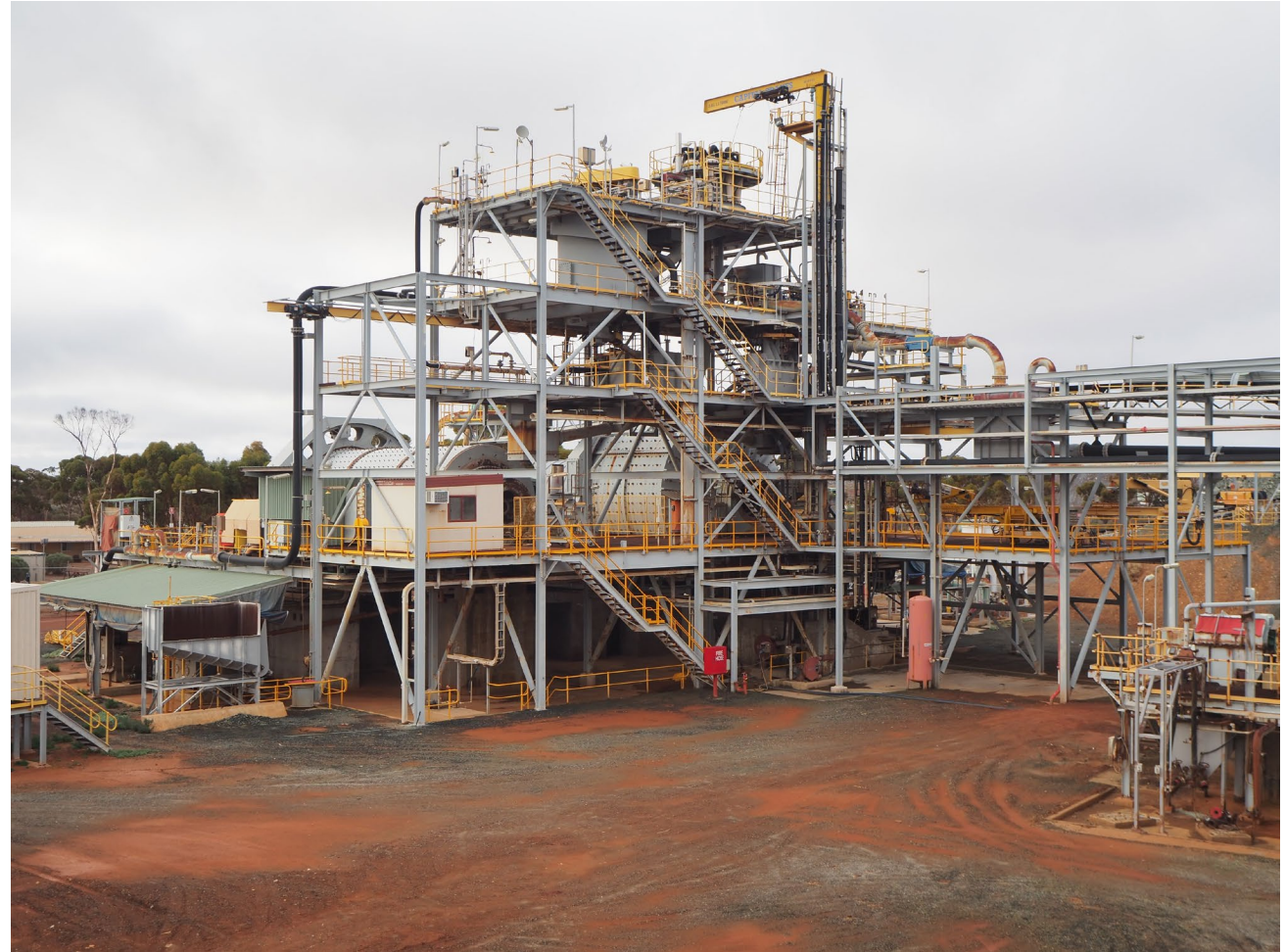
Black Swan Grinding Circuit and Flash Flotation
