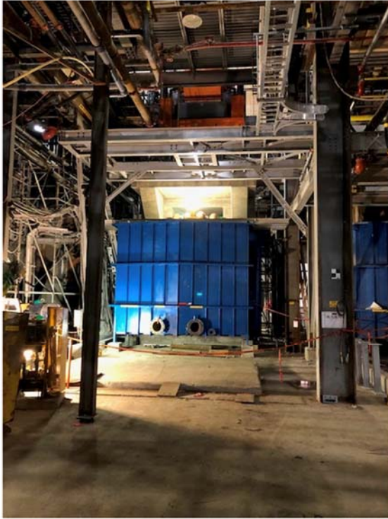
Left: WHIMS installation in preparation for piping; Right: Filter press positioned for concrete pour and installation
