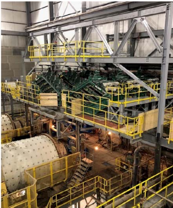
Left: Derrick Screens ready for electrical installation; Right: Conditioning tank in place for full installation
