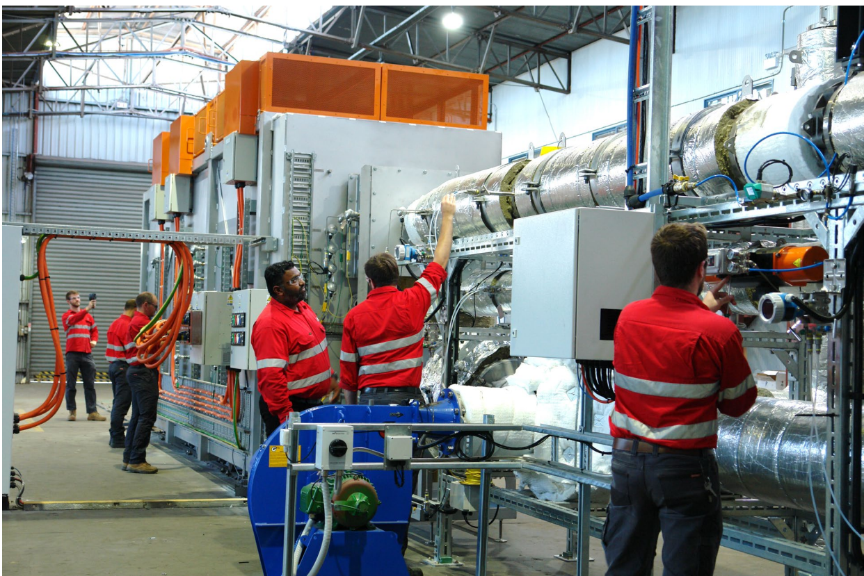
SiBox Demonstration Module on track
