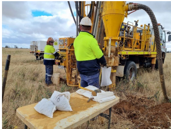
Figure 1 - Wallis contractors during December 2022
