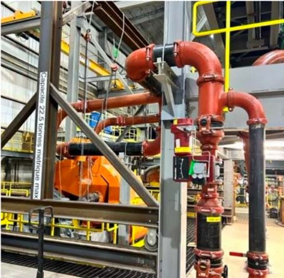
WHIMS rubber-lined piping installation (left); gate valves (right)
