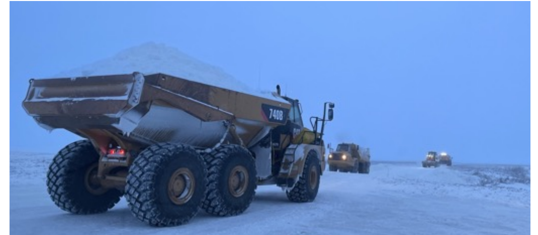
Ice road construction
