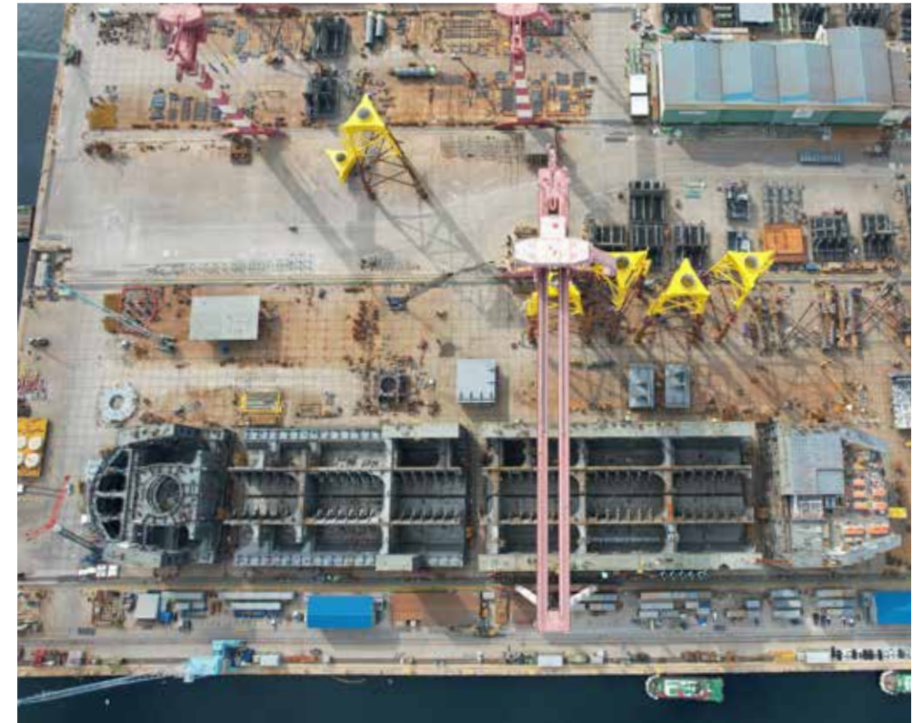
Barossa FPSO construction
