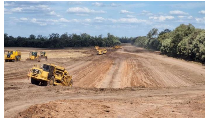
Irrigation channel supporting 4,000 ML water storage under development. Baamba Plains, November 2022.
