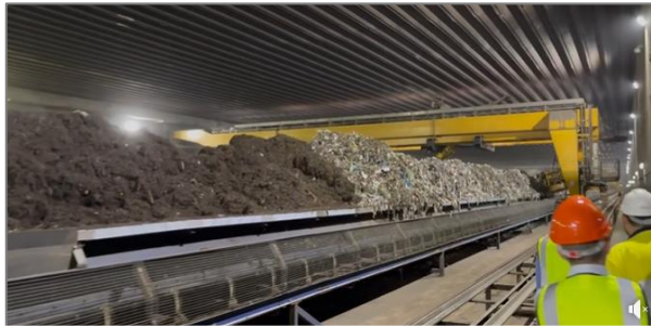
Composting hall at GRL during FOGO trial
