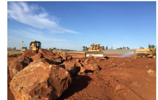
Maas Civil project site
