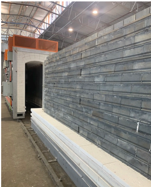
14D BRICK wall in the SiBox Demonstration Module
