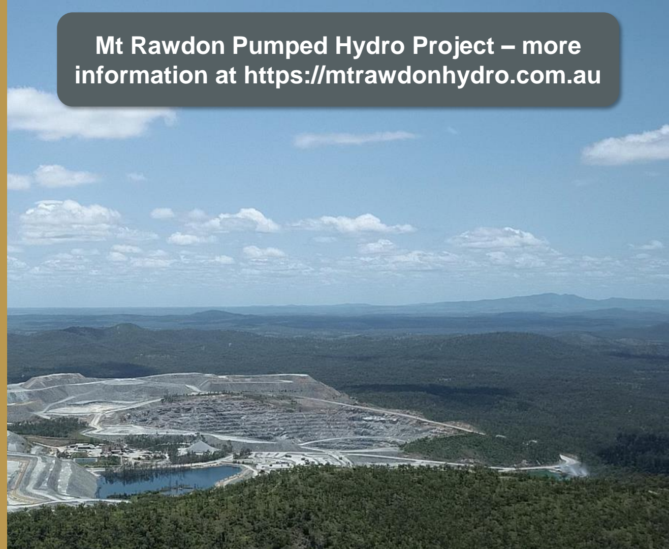
Proposed upper dam area looking down to Mt Rawdon open pit (lower reservoir)
