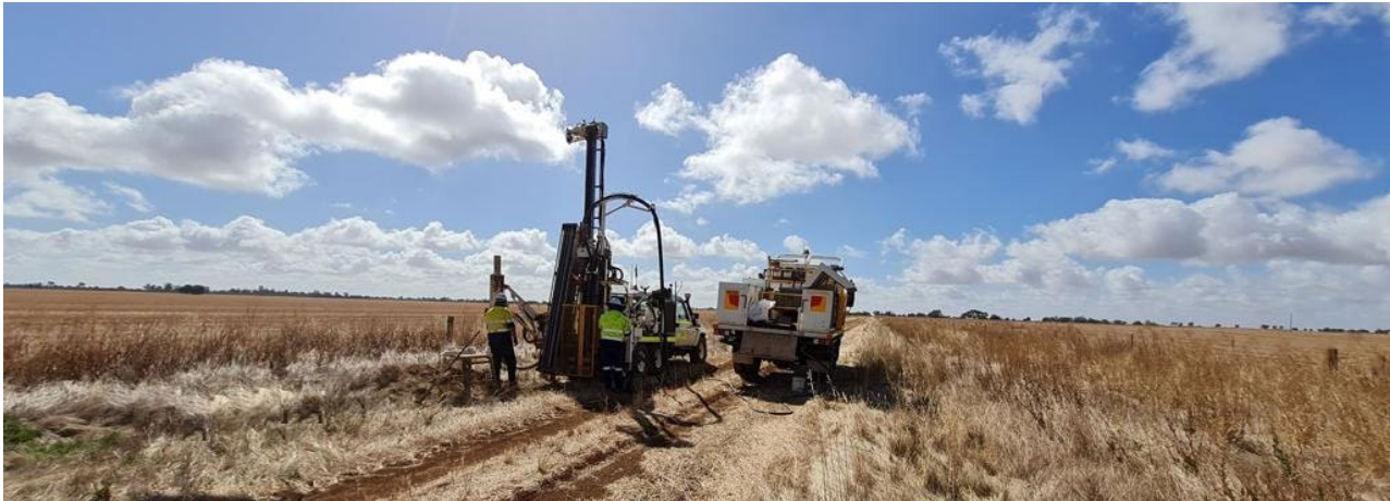
Figure 2 - Wallis contractors during February 2023 at Goschen Central Project
