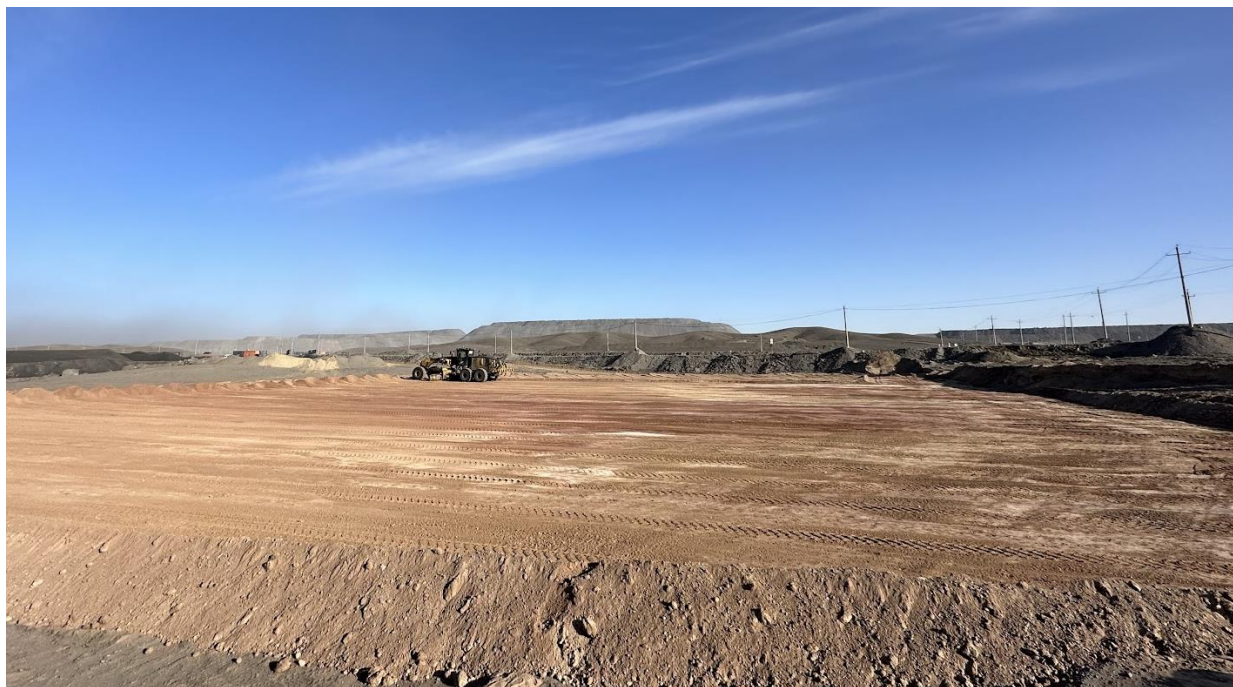
Figure 3 - Preparing Drill Pad for PW-2
