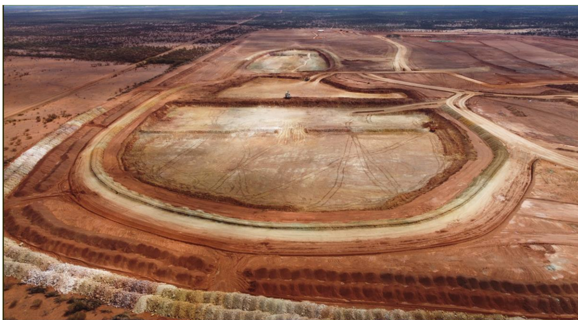
Figure 3: Ben Hur southern pit progress
