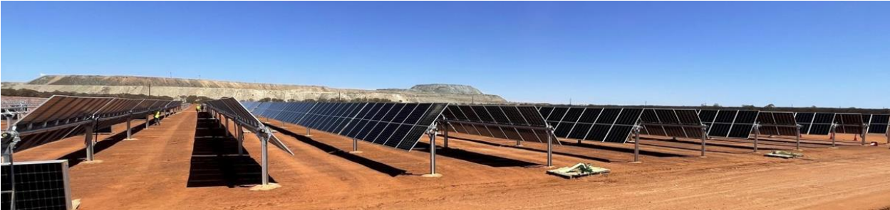
Figure 1: Installation of the 9MW solar farm at Duketon South
