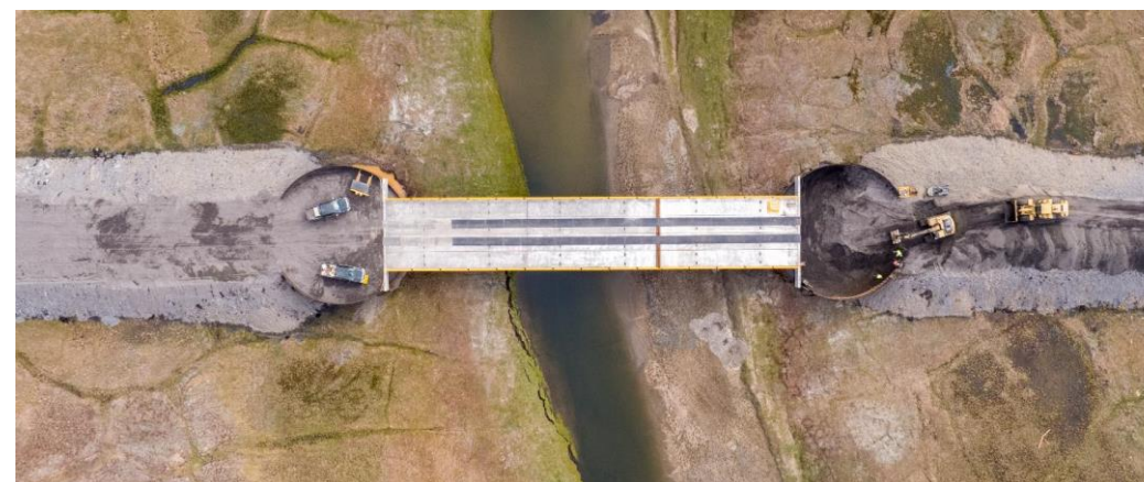
Gravel work completed in 2020/21.
