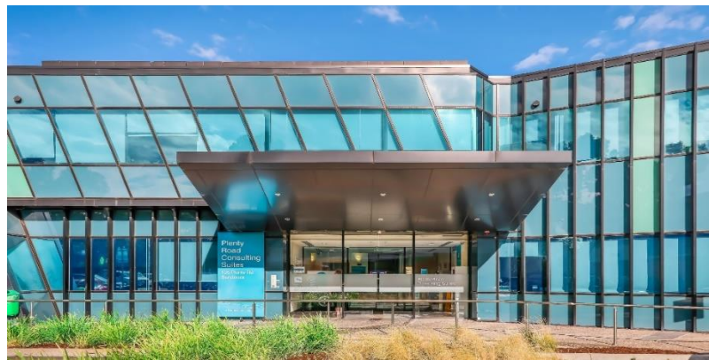
Northpark Private Hospital
