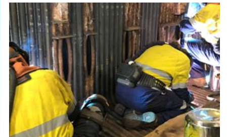
BOILER TUBE LEAD REDUCTION PROGRAM
