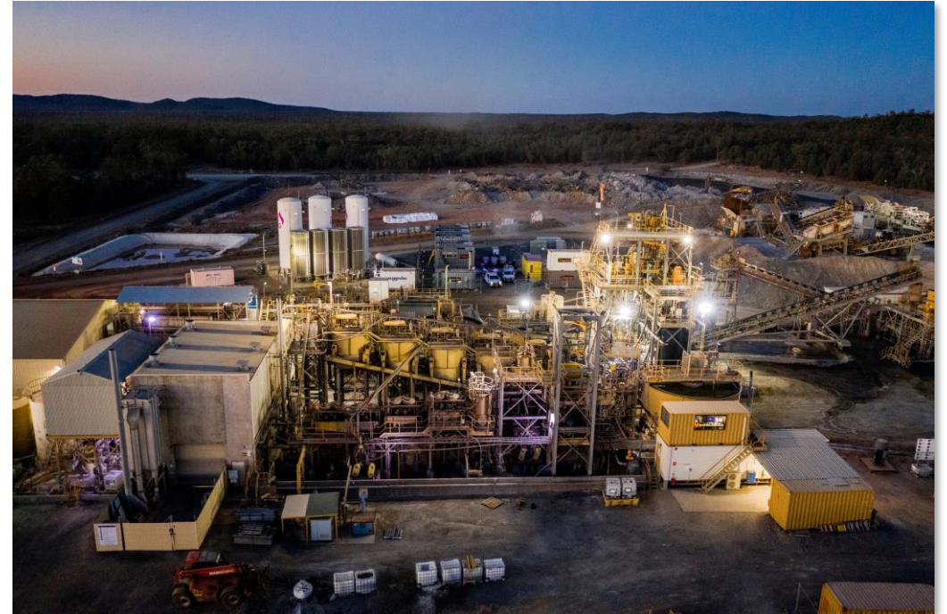
Hera Processing Facility
