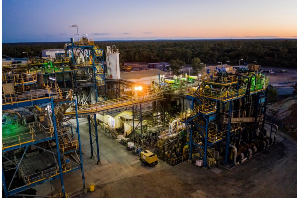
Peak Mine Processing Facility
