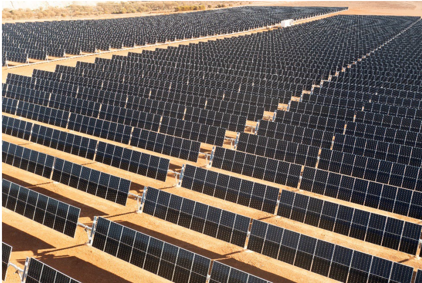
Figure 1: Installation of the 9MW solar farm at Duketon South
