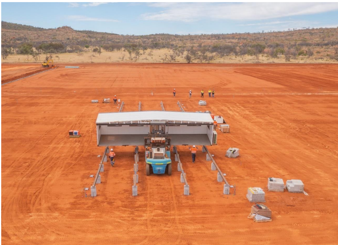
Figure 2: Installation of the first floor of the Nolans construction camp mess buildings, May 2023
