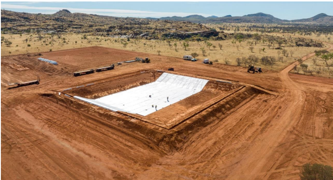
Figure 5: Construction of the site raw water storage dam in progress, June 2023
