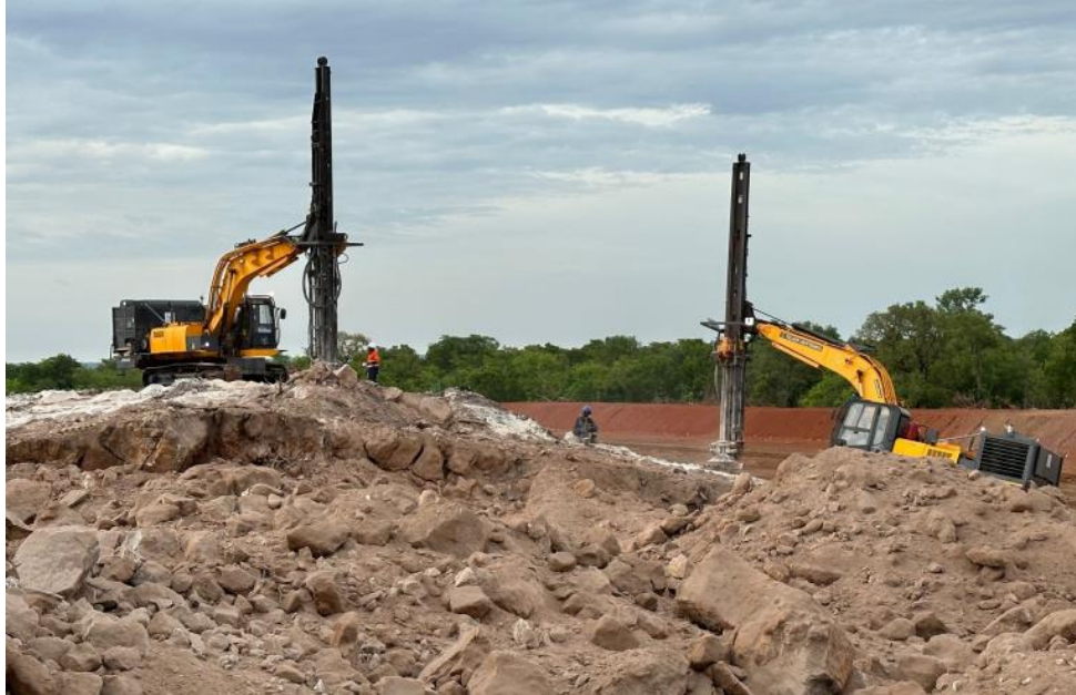
Image 6 - Mining contractor mobilised initial fleet.
