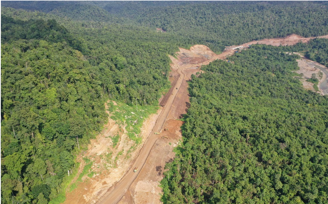
Aerial image of haul road route
