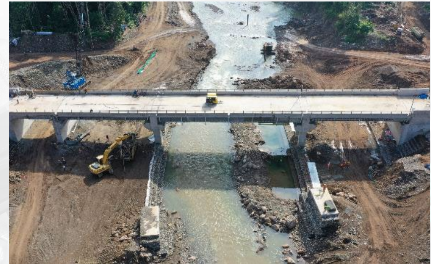
Haul road bridge now complete
