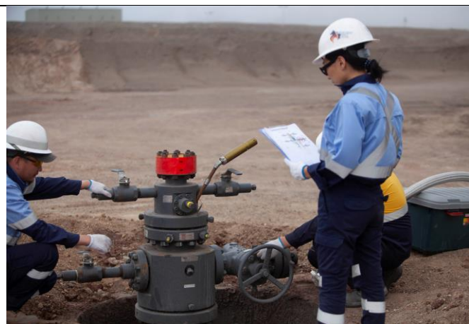
Figure 6 – Preparation for pump and drive head installation at Lucky Fox -3
