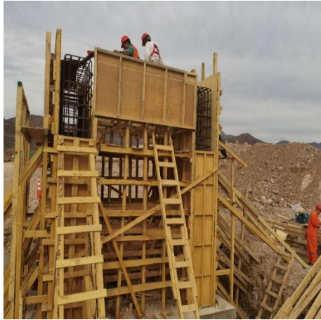
Foundation for the Crushing Machines
