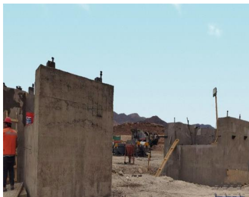
Foundation for the Two Ball Mill Machines
