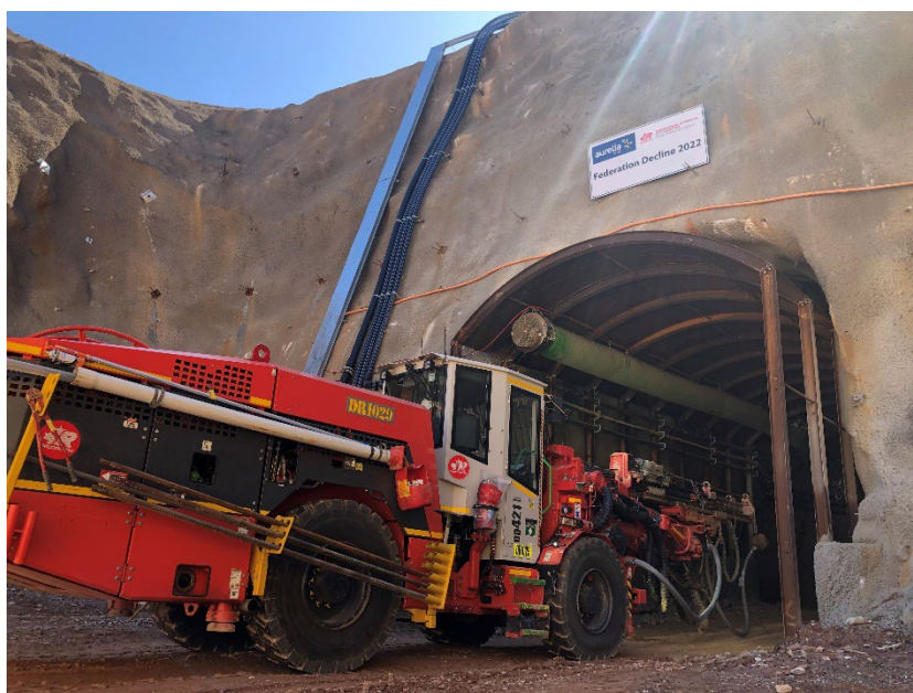
Figure 1: Jumbo tramming into the portal at the Federation Project
