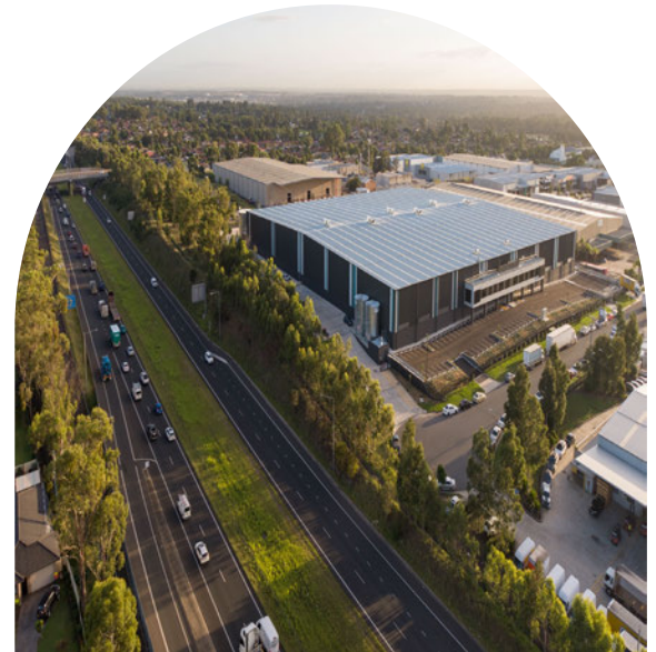
42 Cox Place, Glendenning, NSW
