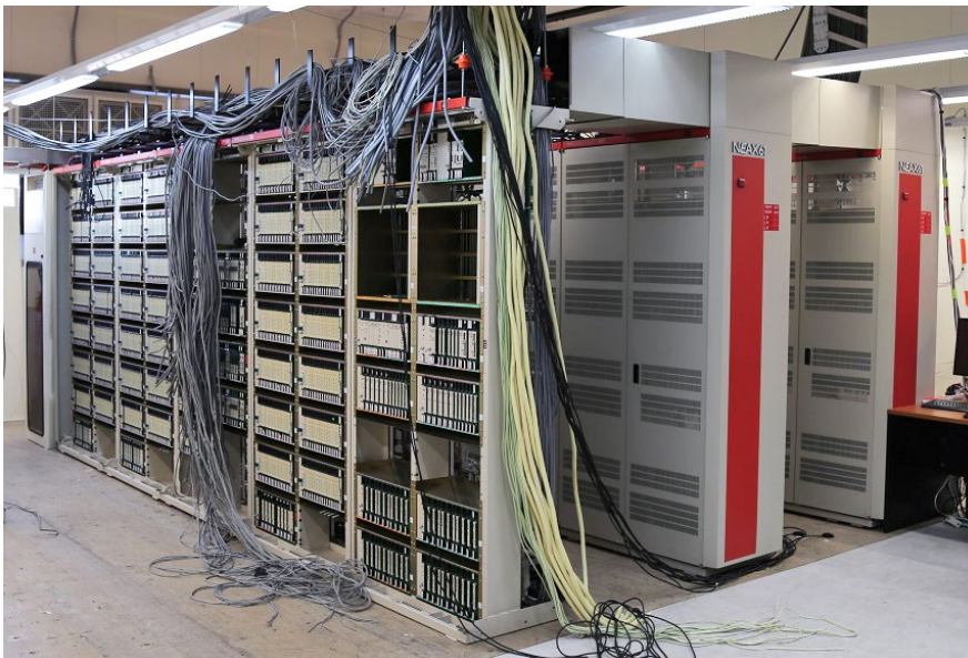
PSTN switches being decommissioned.
