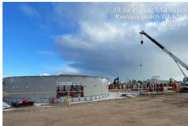
Silo A and B pre-assembly in progress
