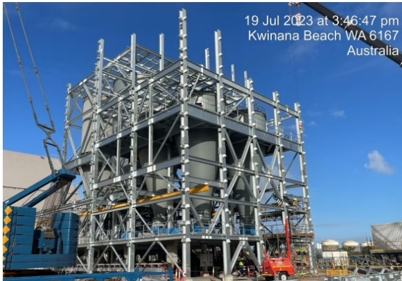
Mill feed building structural works are 37% complete
