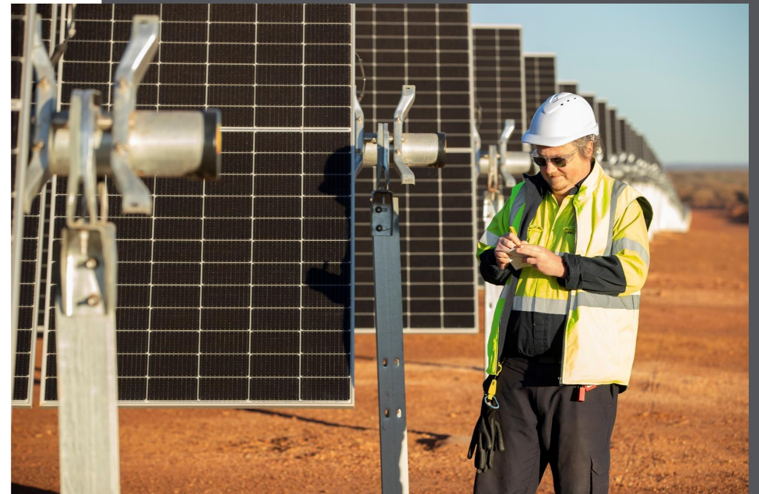
9MW solar farm (Duketon)
